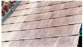
The use of power tools for cutting, drilling, grinding, sanding or sawing asbestos containing material can release significant numbers of fibres as can the use of high pressure water blasters to clean the material prior to painting. These activities must not be performed.
